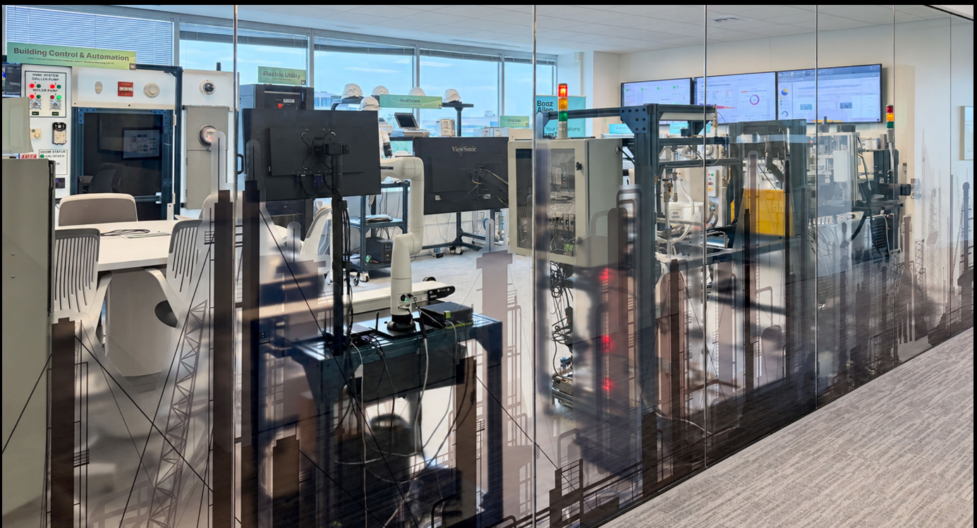
Booz Allen's OT Cybersecurity Lab in Chantilly, Virginia, where the testing was conducted.
